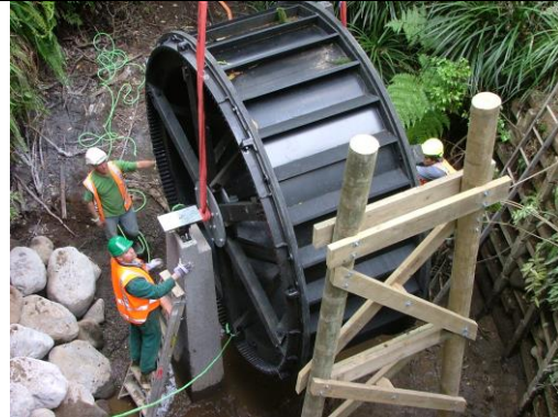
3.6m wheel mounted on two bearings also connected a gearbox and Smart Drive PMA
